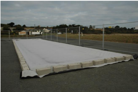
Photo: Bunded watertight platform
