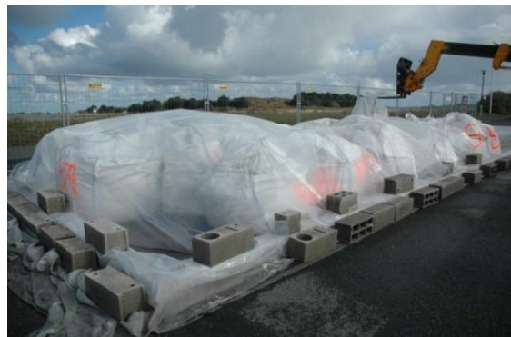
Photo: Cover of a primary storage site with plastic sheet
