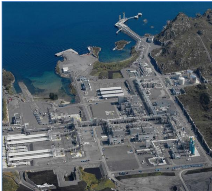
Ormen Lange Gas receiving terminal,
